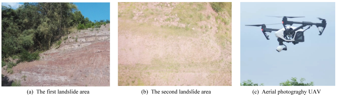
Fig. 9 Field investigation and information collection by UAV
